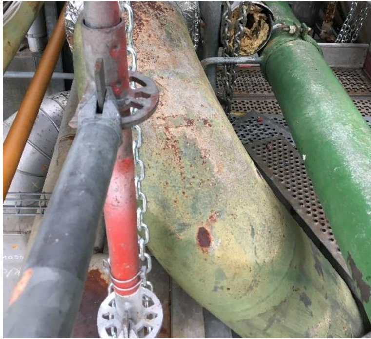
Figure 4: Typical older chemical facility. Tests on this piping revealed had the following result: Difference (Non-Invasive – Invasive): Accuracy (Mean) = +0,14°C, Repeatability (Stdev) = 0,13°C
